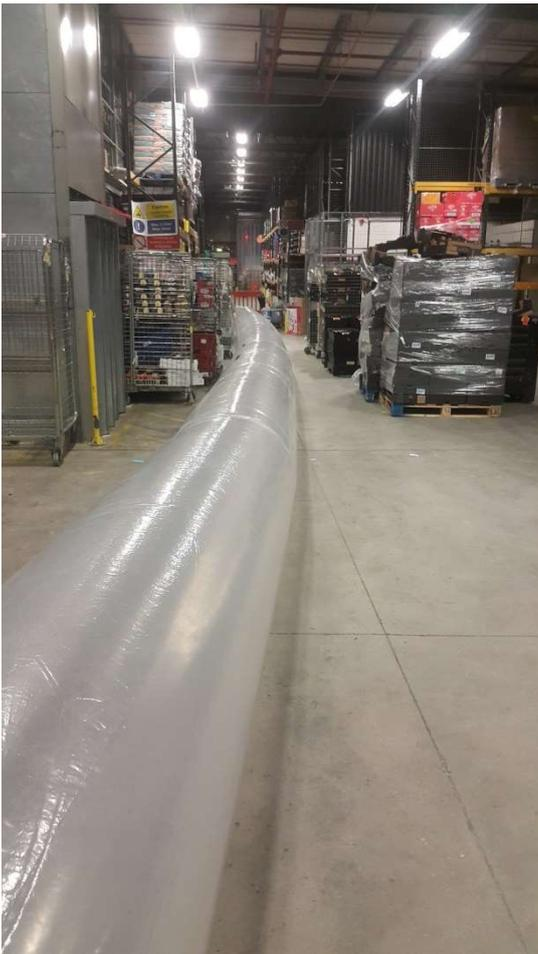
The vapours are vented out of the building using large fans connected to 1m diameter plastic tubing with more fans blowing air towards the exit as shown above.
