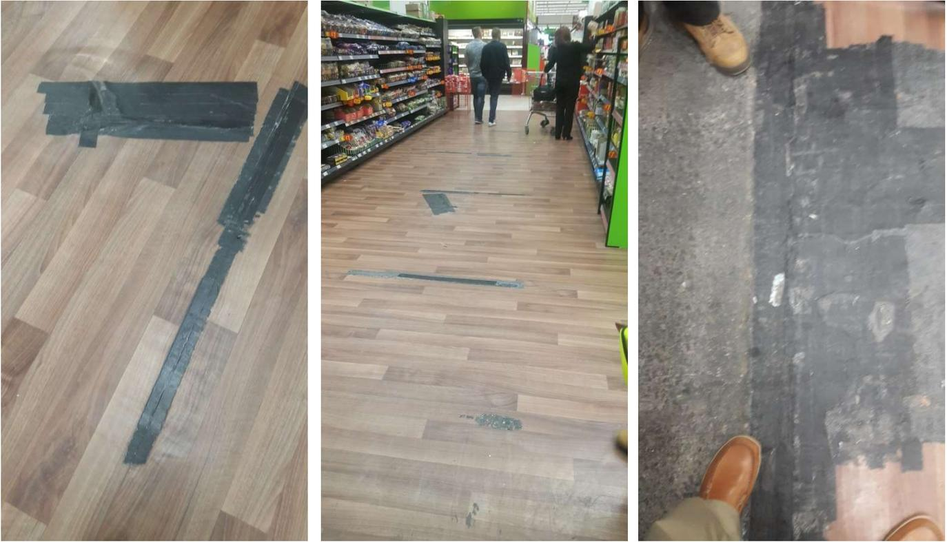
Pictures show the extent of the damaged floor that was both unsightly and a trip hazard to staff and shoppers. This is the main gangway from the warehouse into the main shop, so is heavily trafficked by product trolleys and staff. Having already replaced the vinyl a couple of times in this area, Asda decided to invest in a hard wearing resin system that could take the abuse.
